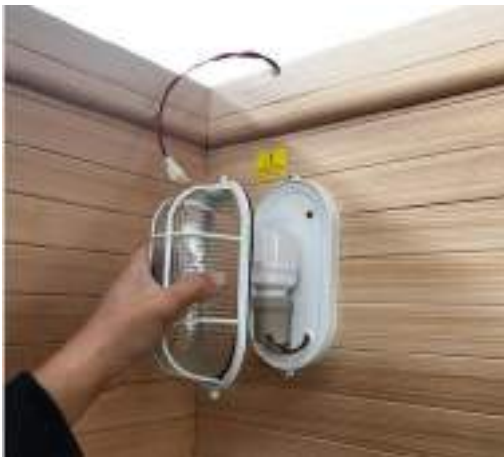
(11) Install sauna lights waterproof cover, just use screws, see above photo the screws is 4x12mm
