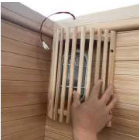
(12) Assemble wood cover for sauna lights 3x25 mm 8 pcs
